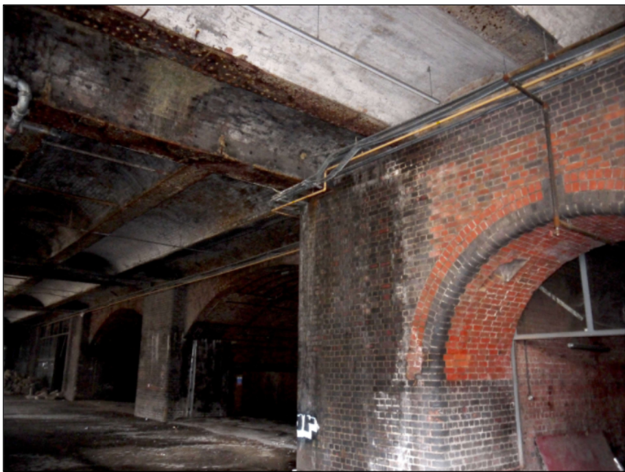
EXAMPLES OF DEGRADATION OF JACK ARCH BEAMS DUE TO WATER INGRESS FROM PARK LEVEL ABOVE - Please see Structural engineers report for description of required remedial works.
