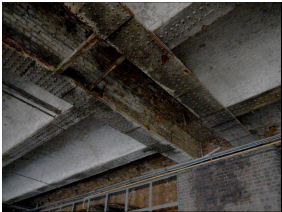
EXAMPLES OF DEGRADATION OF JACK ARCH BEAMS DUE TO WATER INGRESS FROM PARK LEVEL ABOVE - Please see Structural engineers report for description of required remedial works.
